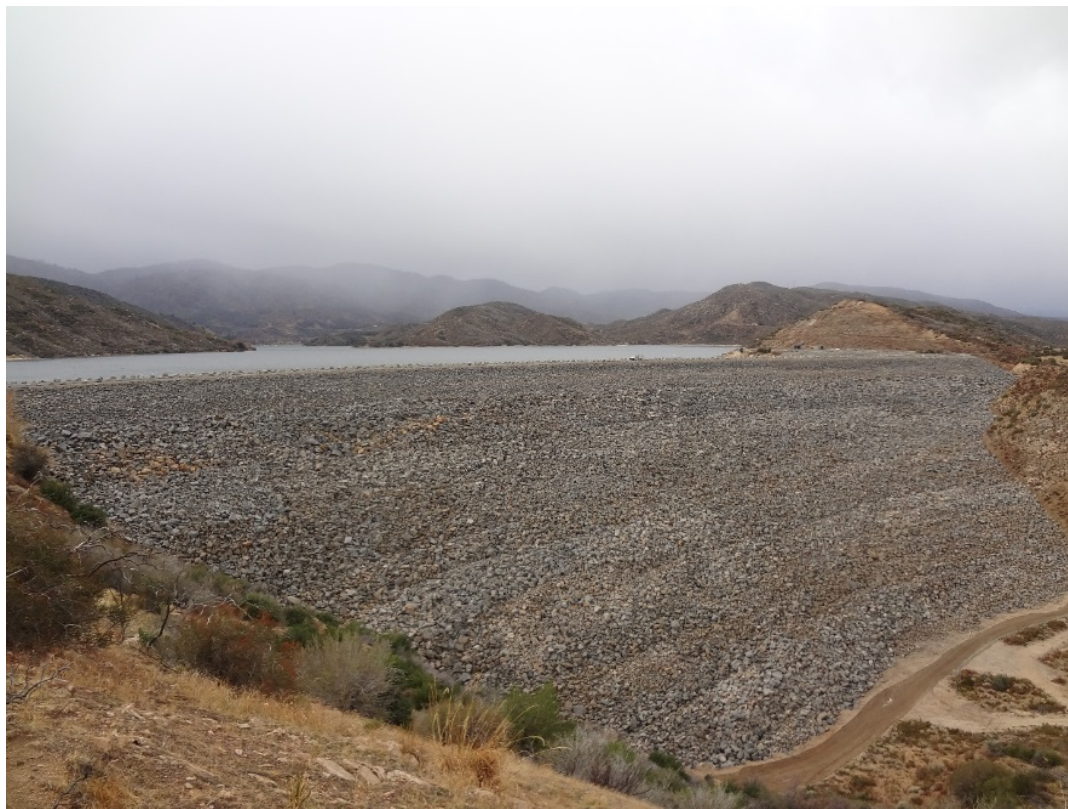
Figure 3.2-1. Downstream Face of Cedar Springs Dam and Silverwood Lake from the Right Abutment
