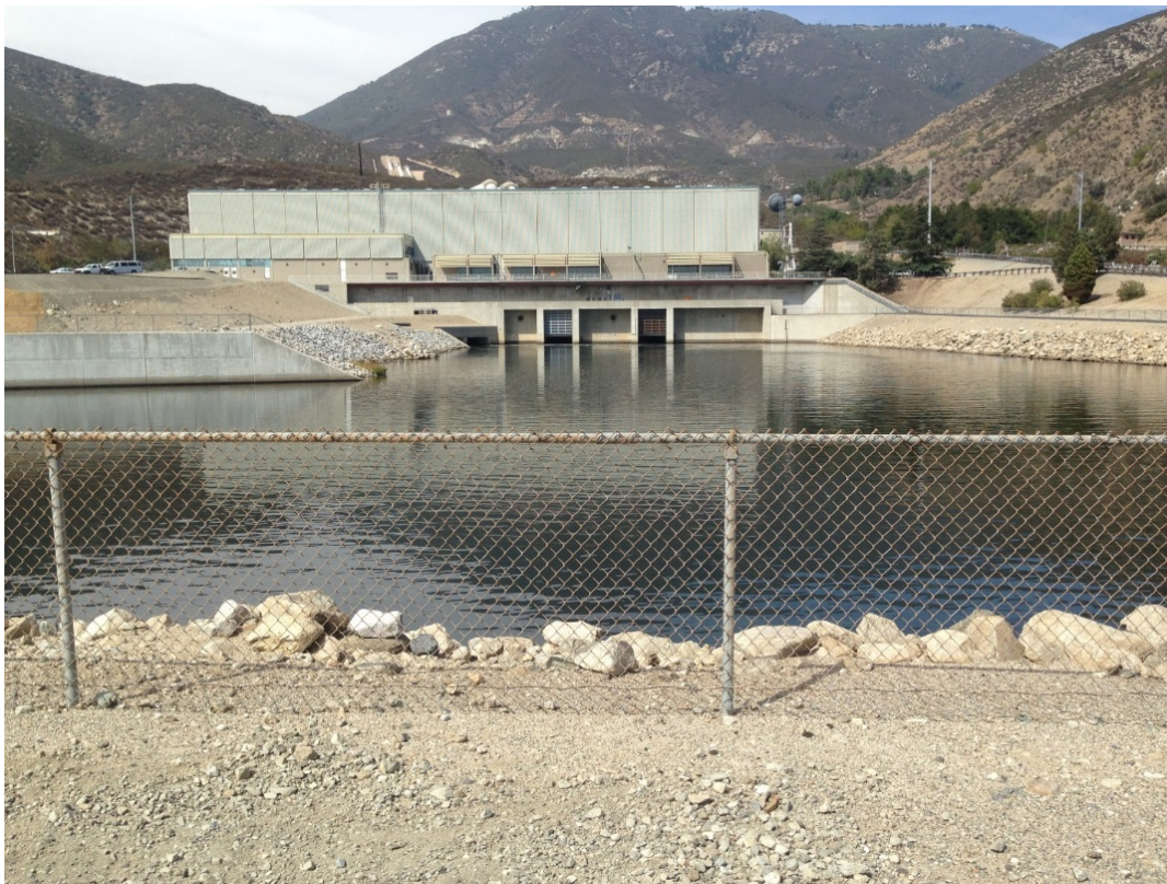
Figure 3.2-2 Devil Canyon Powerplant and Devil Canyon Afterbay from the Road Leading to the Second Afterbay
