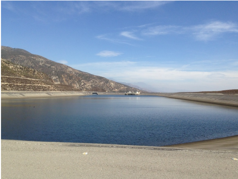
Figure 3.2-3. Devil Canyon Second Afterbay from the West Side of the Afterbay
