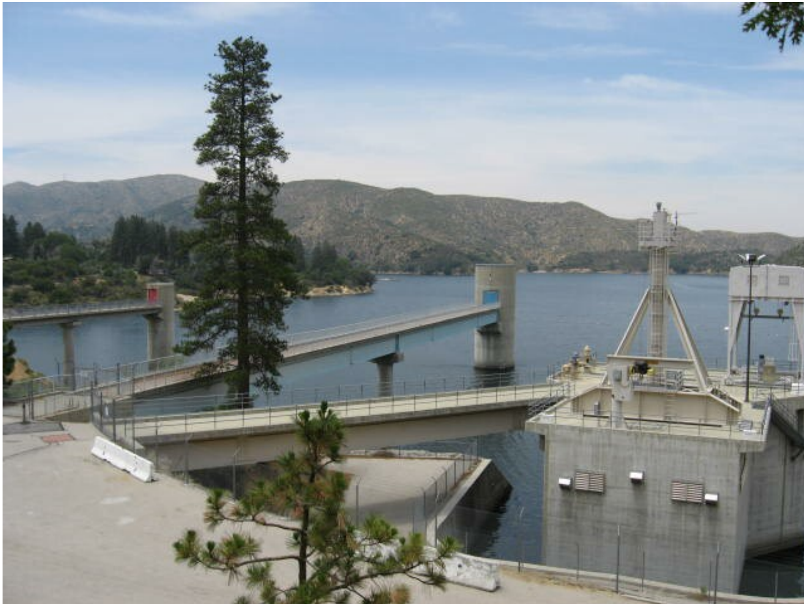
Figure 4.10-10. Silverwood Lake Outlet Area (2009)
