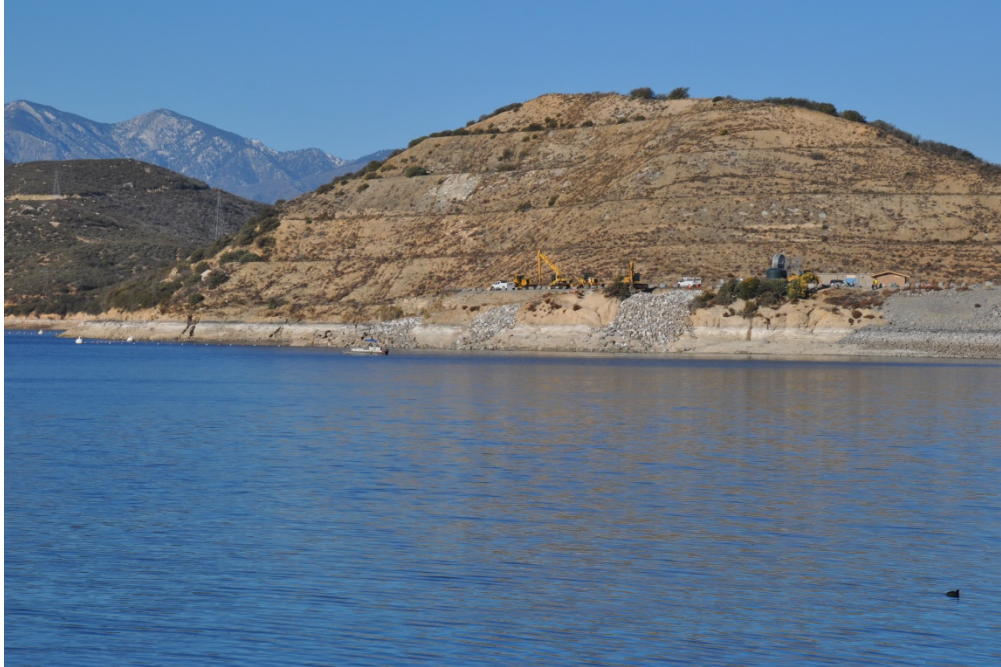
Figure 4.3-7. 2015 Erosion and Stabilization Repair
