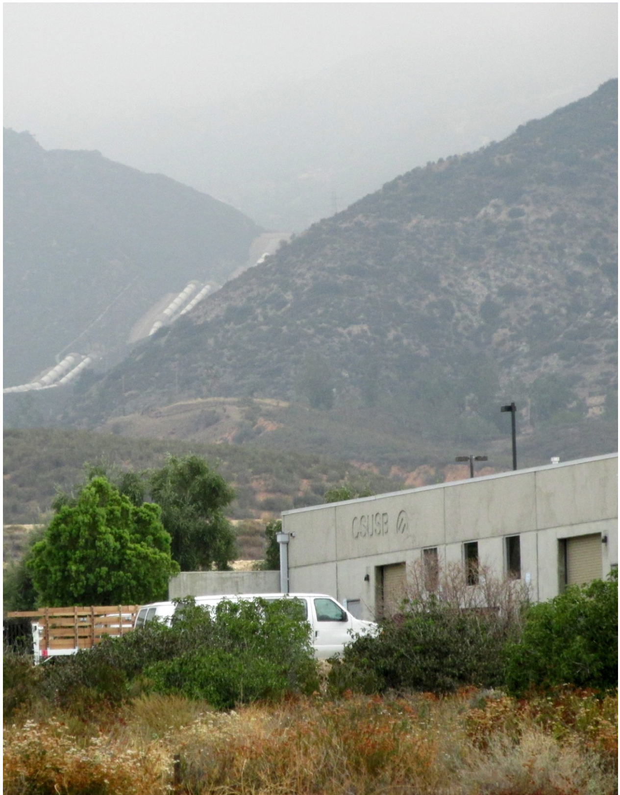
Figure 4.10-14. Devil Canyon Powerplant Penstocks from CSUSB Campus (2015)
