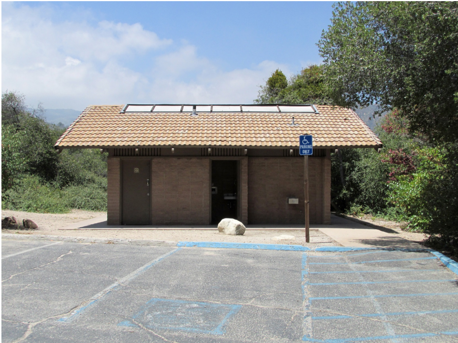
Figure 4.9-14. New Mesa Campground Comfort Station (2015)
