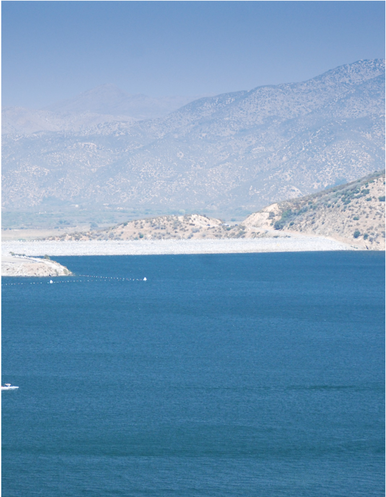
Figure 4.10-2. Cedar Springs Dam from Silverwood Lake (2015)
