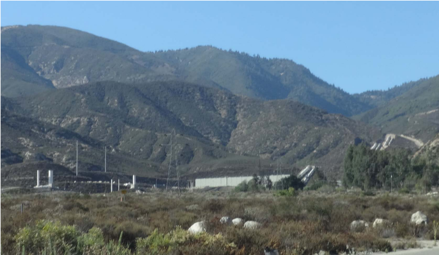
Figure 4.10-13. Devil Canyon Powerplant as seen from Devil Canyon Road (2015)
