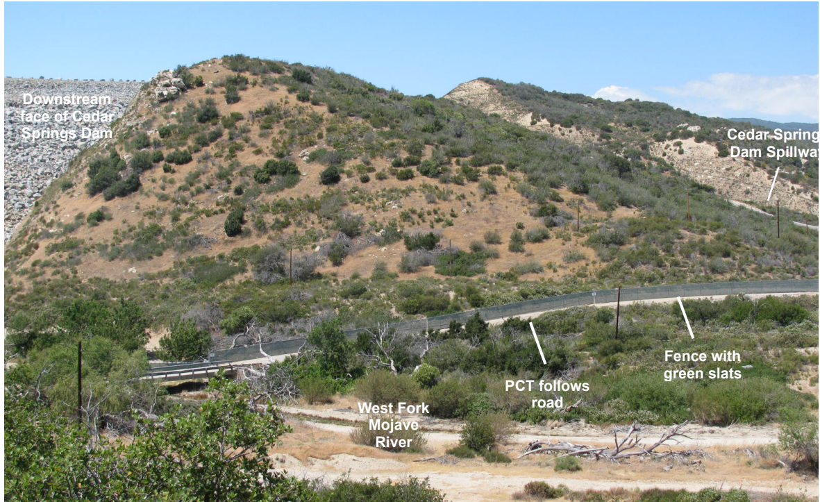
Figure 2.1-2. Fence with Green Slats Along the PCT as Viewed from the PCT Along the Ridgeline as the Project is First Viewable by PCT Users from the North
