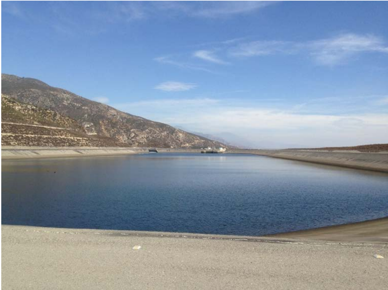
Figure 3.6-1. Devil Canyon Second Afterbay from the West Side of the Afterbay Looking East
