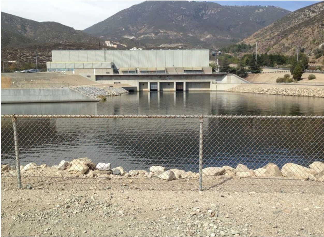
Figure 3.3-1. Devil Canyon Powerplant and Devil Canyon Afterbay from the Road Leading to the Second Afterbay
