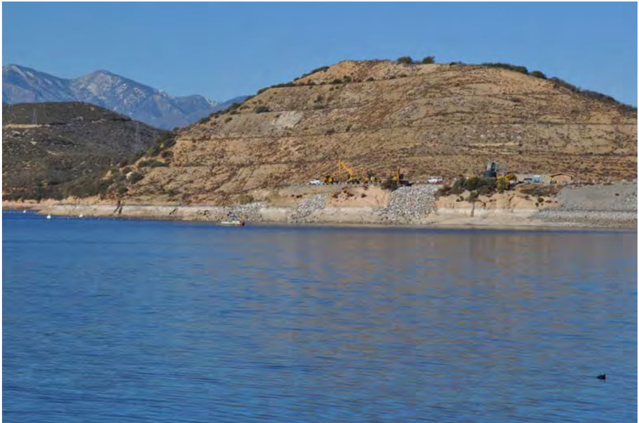
Figure 5.1-7. 2015 Erosion and Stabilization Repair of Silverwood Lake Shoreline
