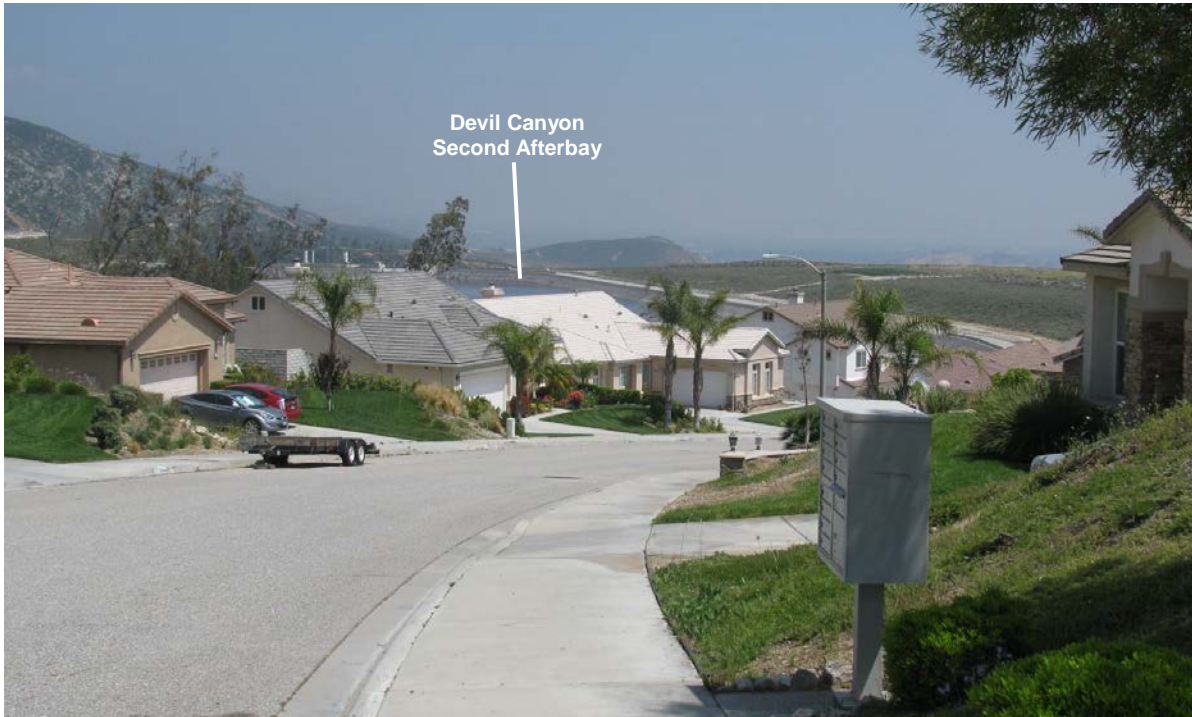
Figure 2.2-4. Devil Canyon Second Afterbay as Viewed from North Melvin Avenue
