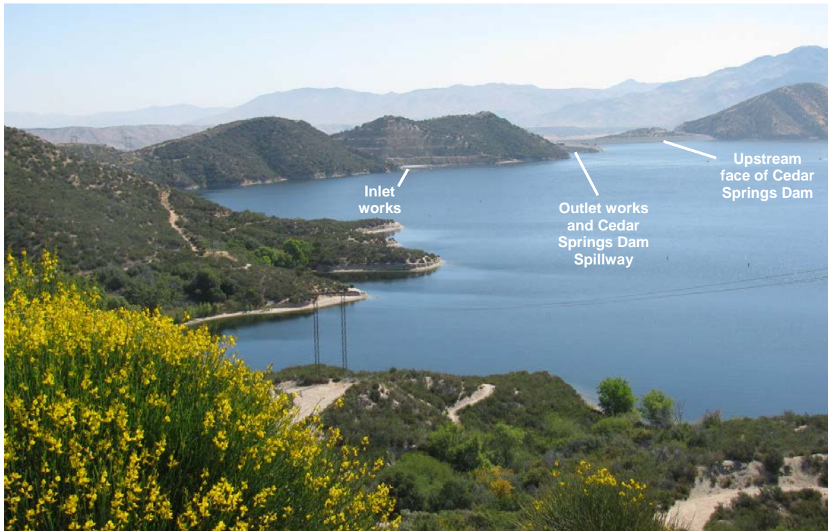
Figure 2.1-5. Cedar Springs Dam and Spillway as Viewed from State Highway 138 from the Reservoir Side
