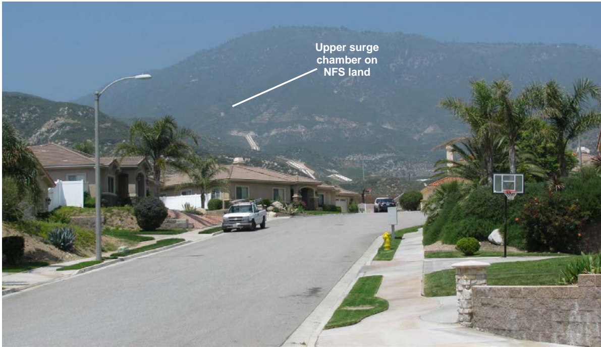
Figure 2.2-1. Devil Canyon Powerplant, Penstocks and Surge Chamber as Viewed from Ohio Street at Ashley Court
