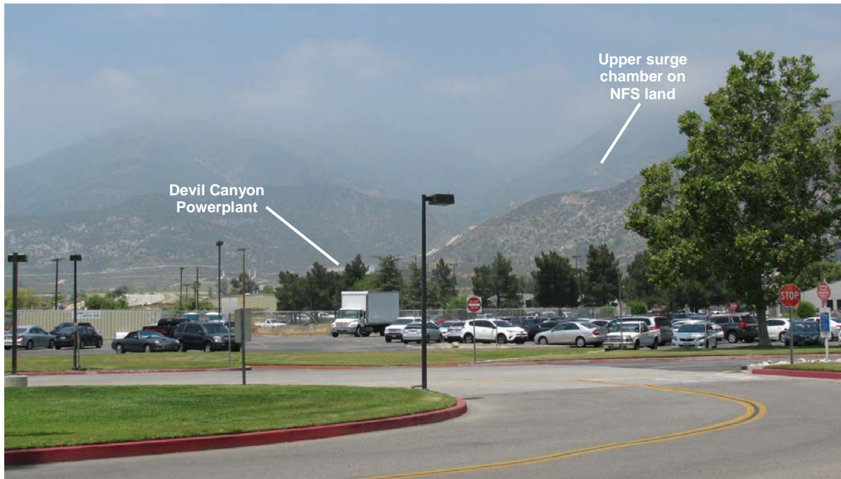
Figure 2.2-3. Devil Canyon Powerplant, Penstocks and Surge Chamber as Viewed from California State University San Bernardino
