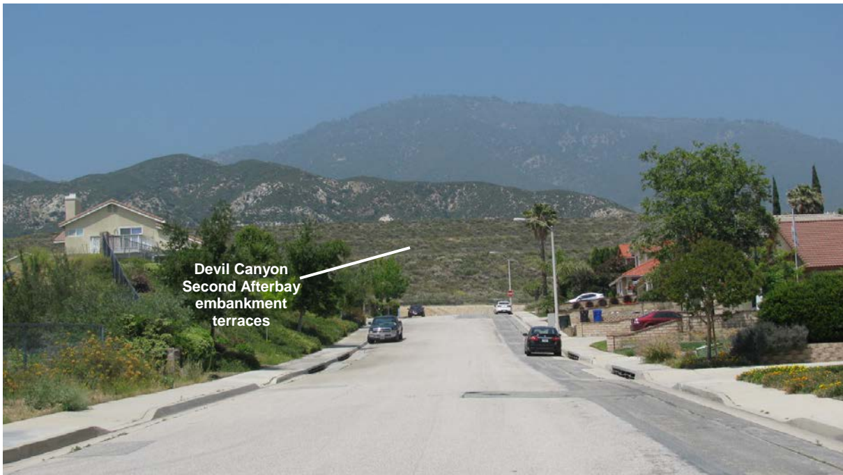
Figure 2.2-5. Devil Canyon Second Afterbay Embankment Terraces as Viewed from North Walnut Avenue
