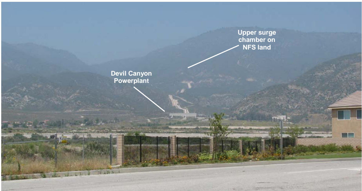
Figure 2.2-2. Devil Canyon Powerplant, Penstocks and Surge Chamber as Viewed from Campus Parkway
