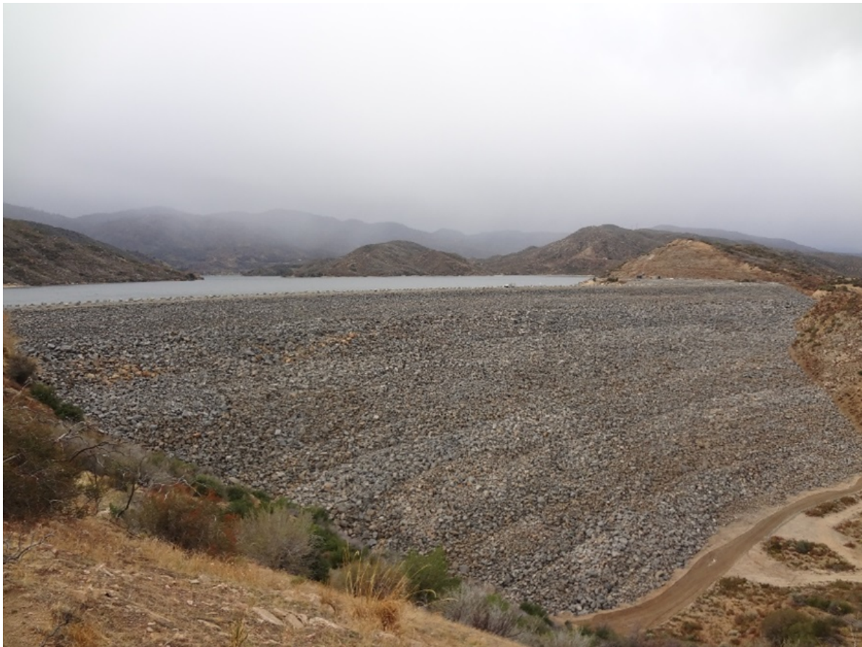
Figure 3.1-1. Downstream Face of Cedar Springs Dam and Silverwood Lake from the Right Abutment
