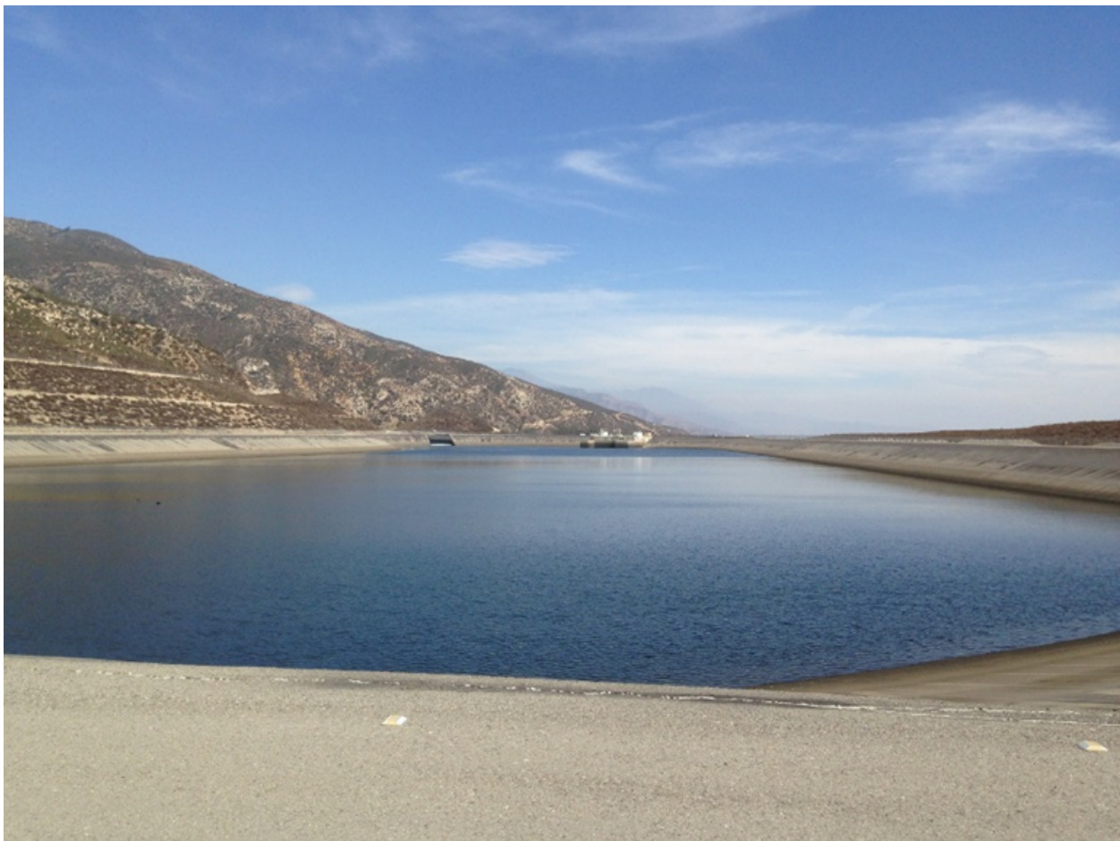
Figure 3.7-1. Devil Canyon Second Afterbay from the West Side of the Afterbay Looking East
