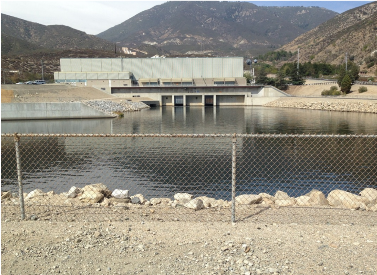
Figure 3.4-1. Devil Canyon Powerplant and Devil Canyon Afterbay from the Road Leading to the Second Afterbay
