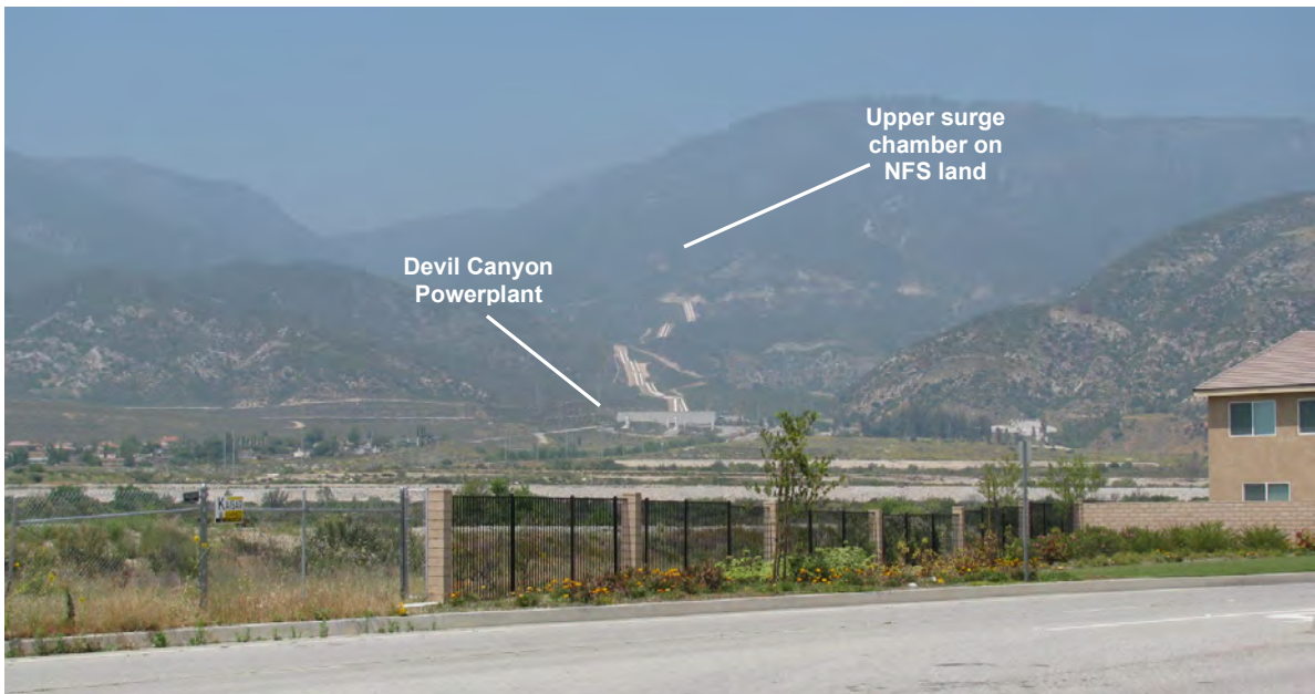
Figure 2.2-2. Devil Canyon Powerplant, Penstocks, and Surge Chamber as Viewed from Campus Parkway
