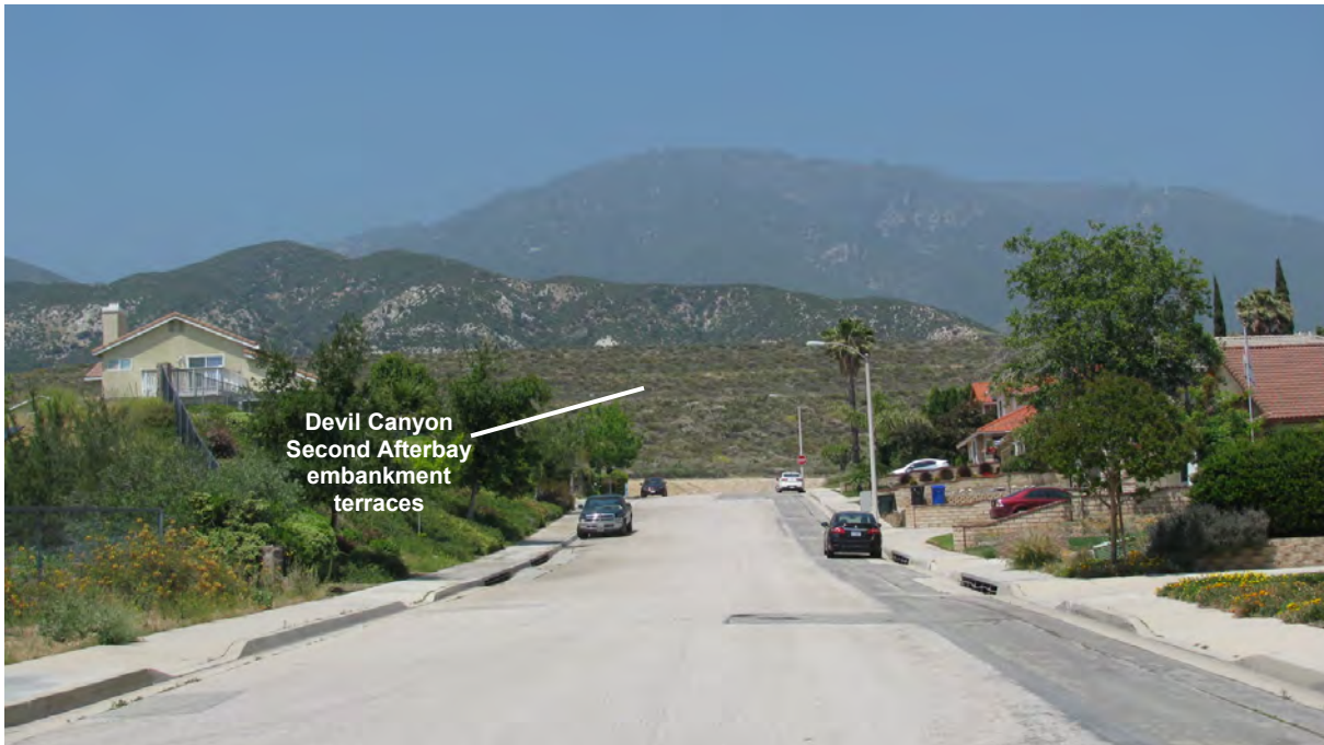
Figure 2.2-5. Devil Canyon Second Afterbay Embankment Terraces as Viewed from North Walnut Avenue
