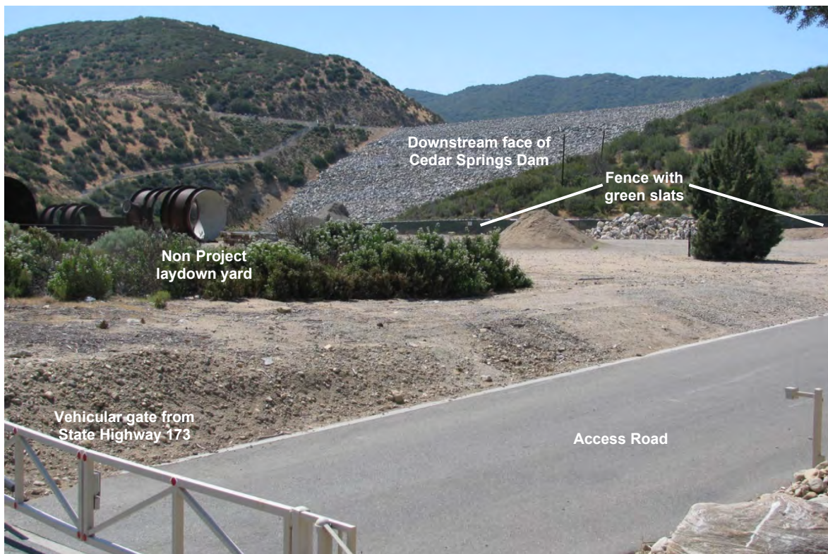
Figure 2.1-3. Cedar Springs Dam as Viewed from the PCT Along The Shoulder of Highway 173 Showing the Fence with Green Slats
