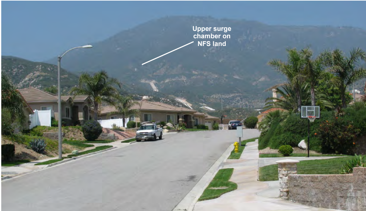
Figure 2.2-1. Devil Canyon Powerplant, Penstocks, and Surge Chamber as Viewed from Ohio Street at Ashley Court
