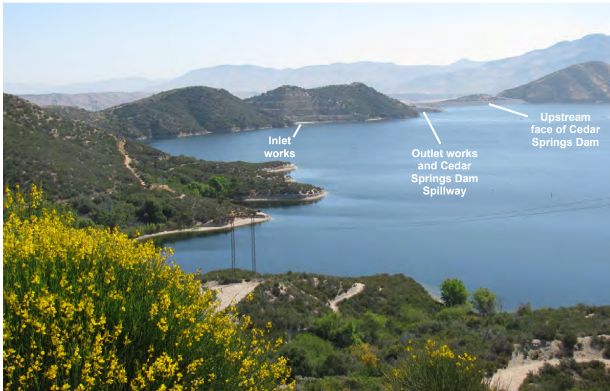
Figure 2.1-5. Cedar Springs Dam and Spillway as Viewed from State Highway 138 from the Reservoir Side
